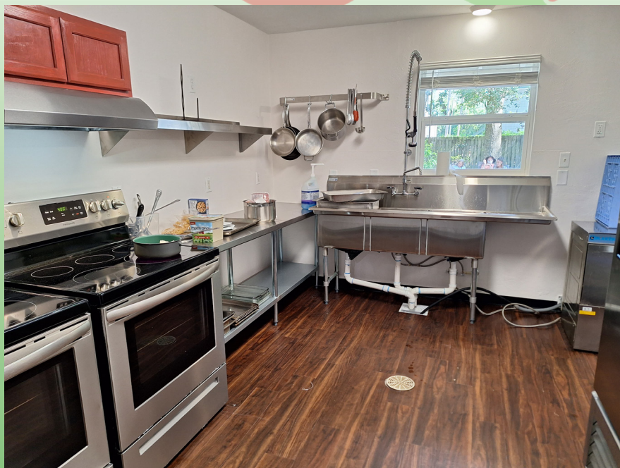
Not only did Rotary donate the money for a kitchen renovation, individual Rotarians donated architectural drawings, contract services, flooring and plumbing. They even negotiated lower prices at contractors rates.
