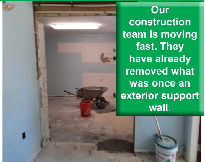
Construction includes partial removal of an exterior wall. This will increase our kitchen size by 50%.
