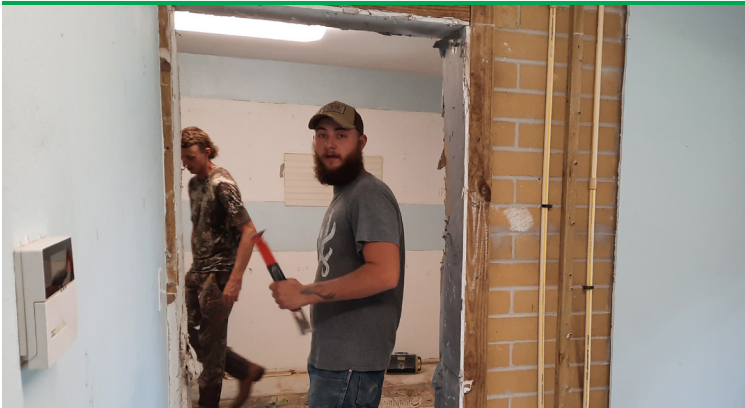
Construction includes partial removal of an exterior wall. This will increase our kitchen size by 50%.
